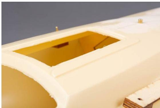
If everything fits, fix the frame with super glue in some places. Then glue the frame with Stabilit Express. Make sure that no glue gets into the side trays for the reinforcement boards of the walls.
